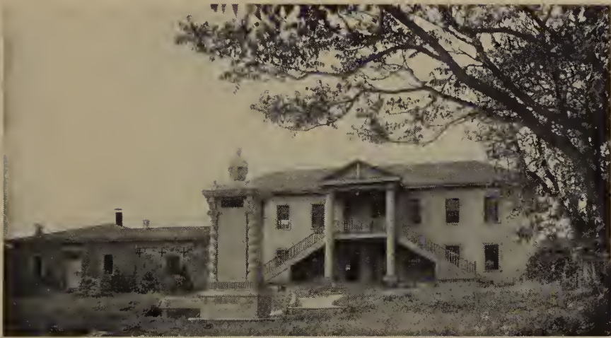
CALIFORNIA'S FIRST CAPITOL BUILDING (Restored), Monterey, California.
